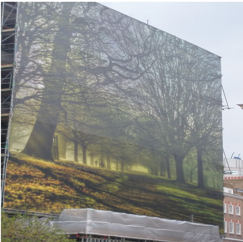
Clever ways of disguising Scaffolding
